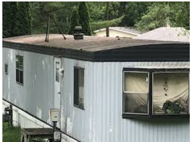
Typical mobile homes at the time came with metal roofs & metal sheet siding.
