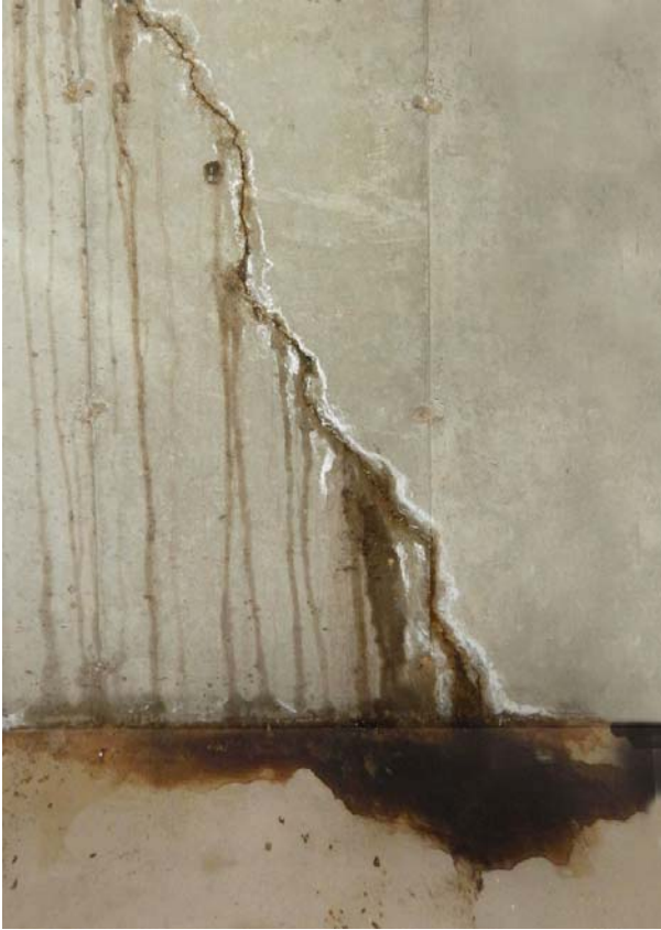
Water can in time heave and damage walls.... actually BOW foundation basement walls
