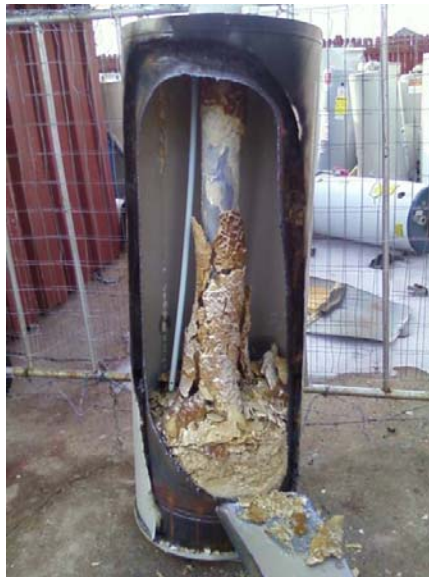
Mineral deposit build-up
