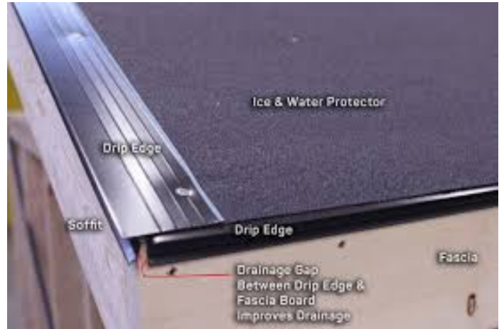
Drip Edge - Inexpensive and easy to install - nails right down.
