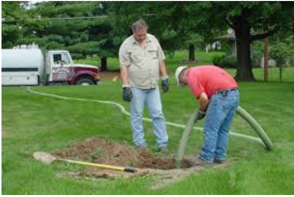
Workers pumping out a home septic tank.
