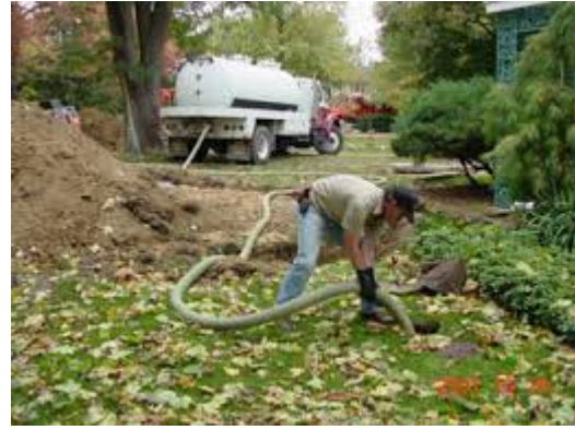
Workers pumping out a home septic tank.
